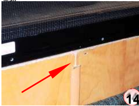
Bottom of window. T-Joiner cut out the same
