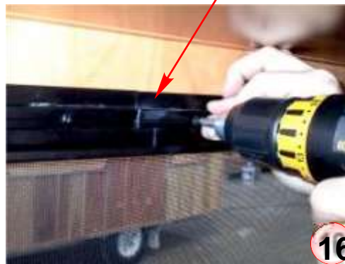
Bottom of window. T-Joiner cut out the same
