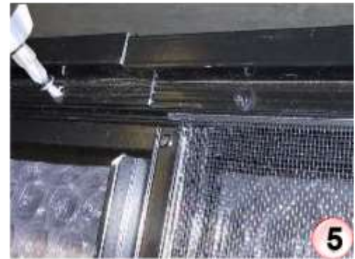
Remove temporary anchoring screws.
